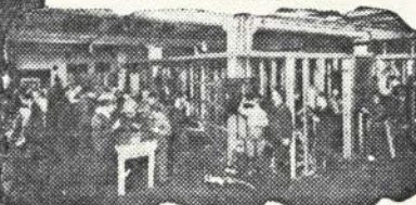
Students Practicing House-wiring In Skeleton Houses
